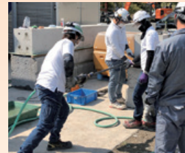
RMA長尺施工
